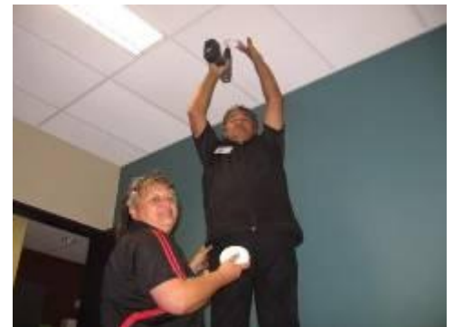
Installation of Smoke Alarms
